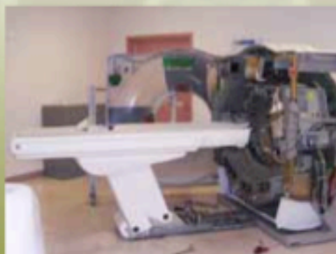
▲ Old CT Scanner being dismantled for removal.
