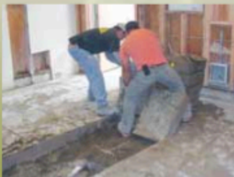
▲ New footings being installed for anchoring of the new CT Scanner.
